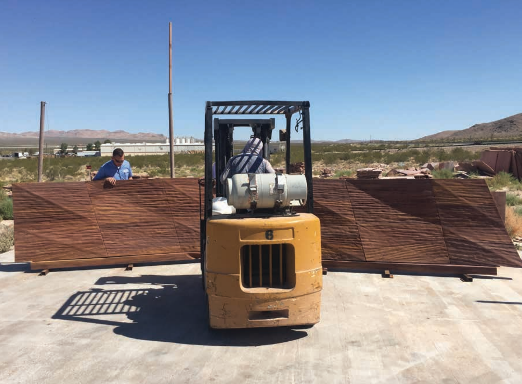
Two mock-ups of the feature wall were also created to ensure color consistency and that the undulated flow was continuous throughout the entire design. Photo courtesy of CORE
